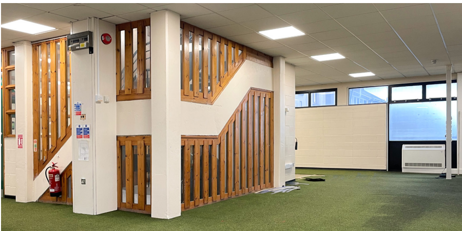
Images below: During refurbishment
